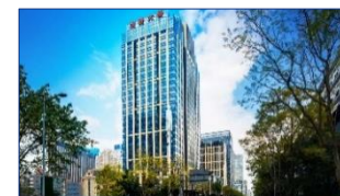
HQ in Chengdu
